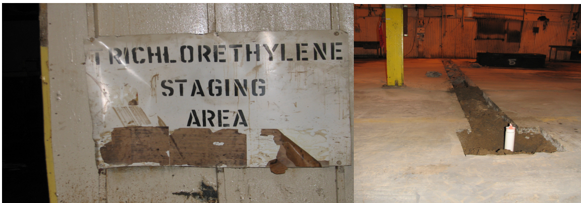
SVE trench and extraction well being installed in background
